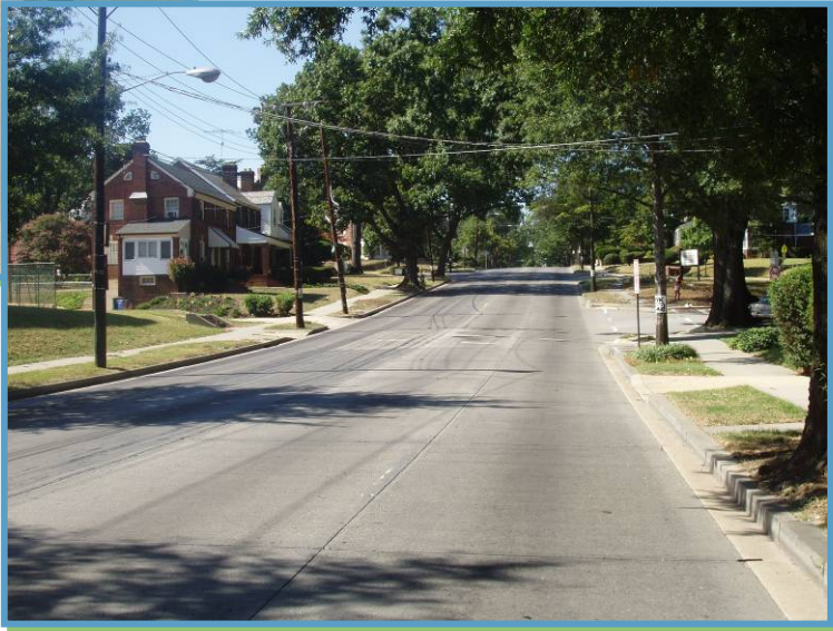
Faded/Missing Pavement Markings along South Dakota Avenue
