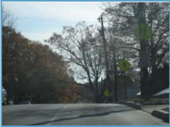
Vertical Alignment Creates Sight Distance Problems
