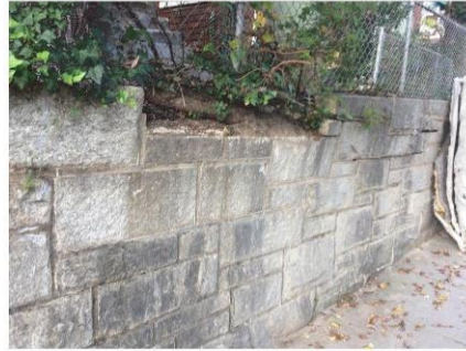
GRANITE BLOCKS REPLACED
