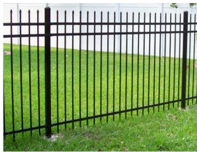
11. 42" HIGH METAL PERIMETER FENCE AT WEST LAWN PARK
