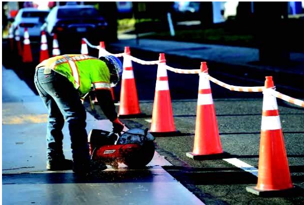
STEP 2: CUTTING & EXCAVATION
