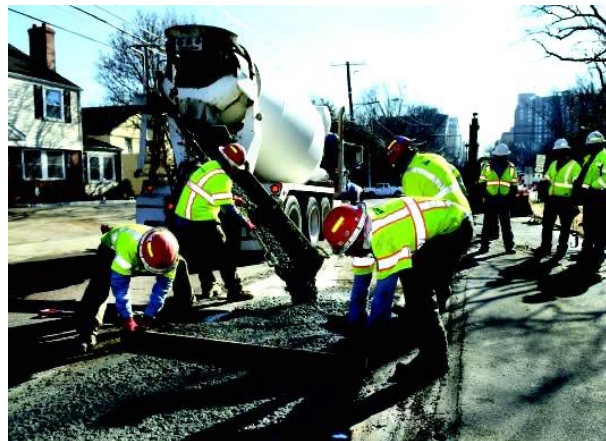
STEP 5: CONCRETE ENCASEMENT
