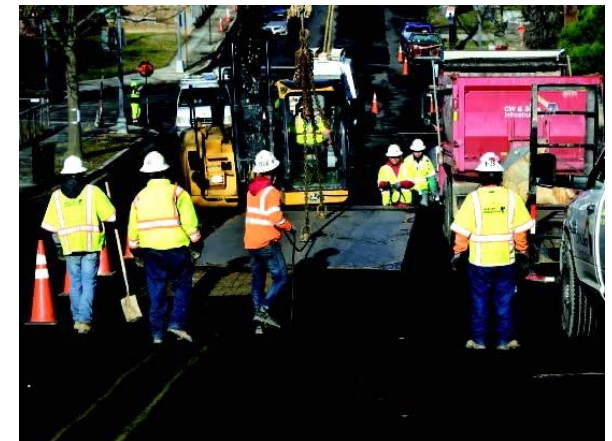
STEP 6: PLATE INSTALLATION, BACKFILLING, & PAVING
