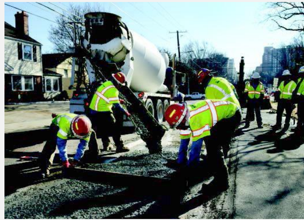
STEP 5: CONCRETE ENCASEMENT
