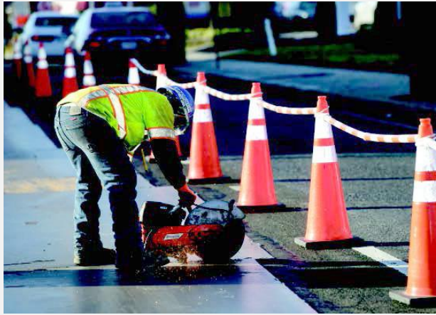
STEP 2: CUTTING & EXCAVATION
